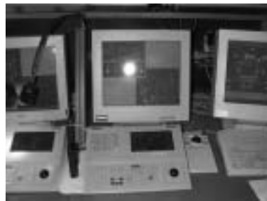
Fig. 4.7. Engine room is moved up on the bridge. From the fast ferry Carisma
